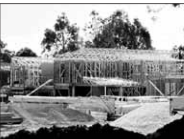
WORK UNDER WAY: Kingfisher Grove, adjacent to the Wetlands Centre.
